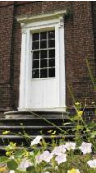
Buckland's gib door empties out onto a 20th century waterfall landing.
